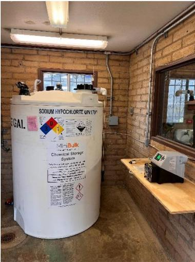
**Chlorine room 405 gallon 12.5% CL<sub>2</sub> storage tank and chemical feed pump.**
