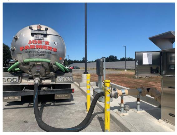
The District and Sonoma Water would require drivers to be fully trained on operation of the transport trucks and the proposed receiving station transfer process. Standard operating procedures to eliminate the potential for leakage during the transfer process is required, including full drainage of connecting hoses prior to disconnection. This Wastewater Receiving Procedure shown below is taped to the inside of the panel door.
