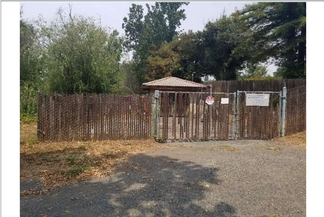
Photo 6. Lift Station 1 Site
