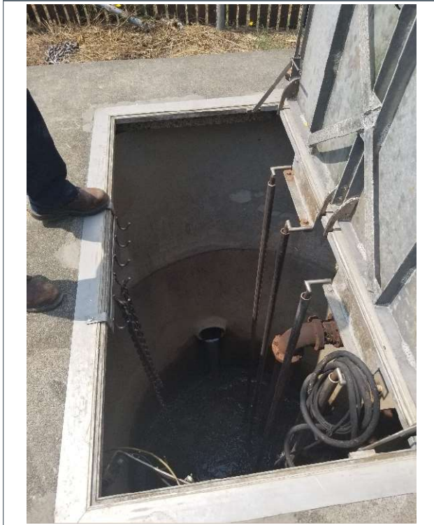
Photo 4. Lift Station 1 Wet Well
